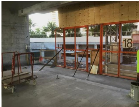
Not installed. Buck hoist.
