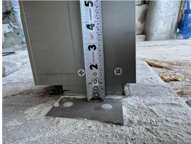
Clip engagement distance of up to 1 9/16”.
