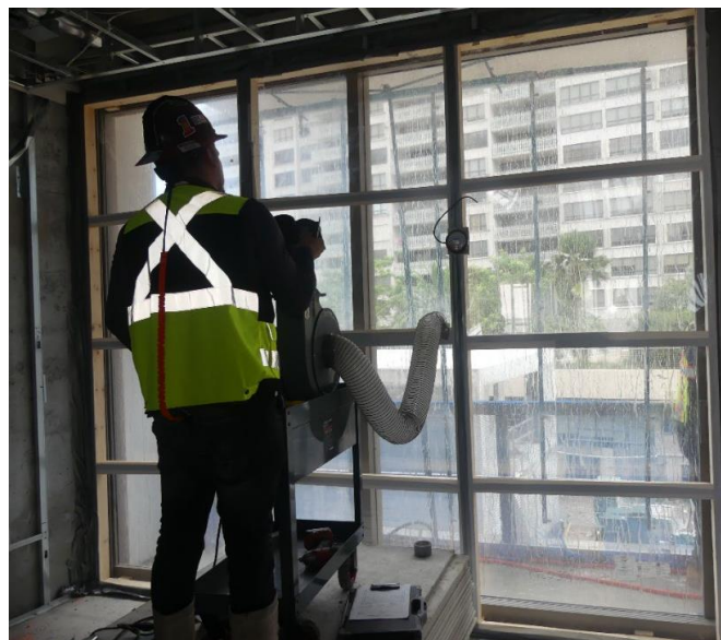
Fig 8: Specimen Being Tested for Water Resistance- Interior View
